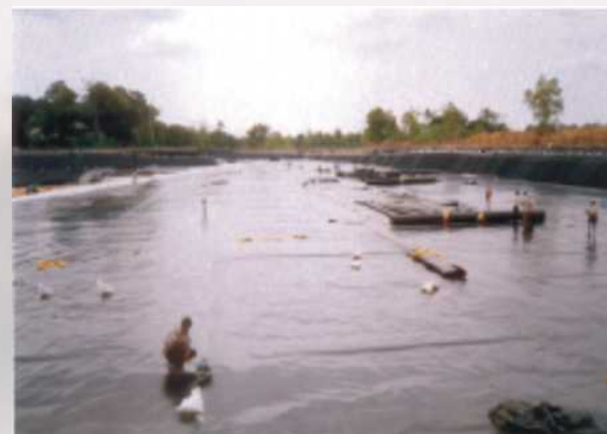
Geomembrane laid on bottom of landfill at Binani Zinc, Cochin.
