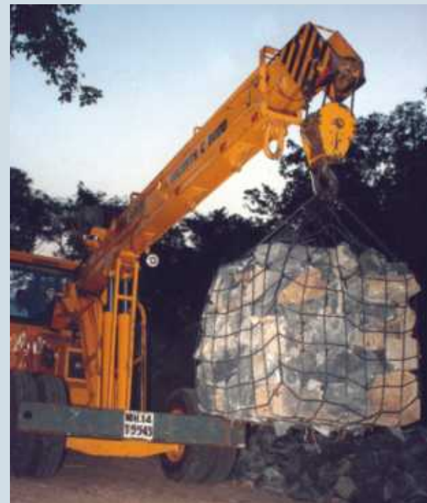
Filled Gabions being lifted for under water installation
