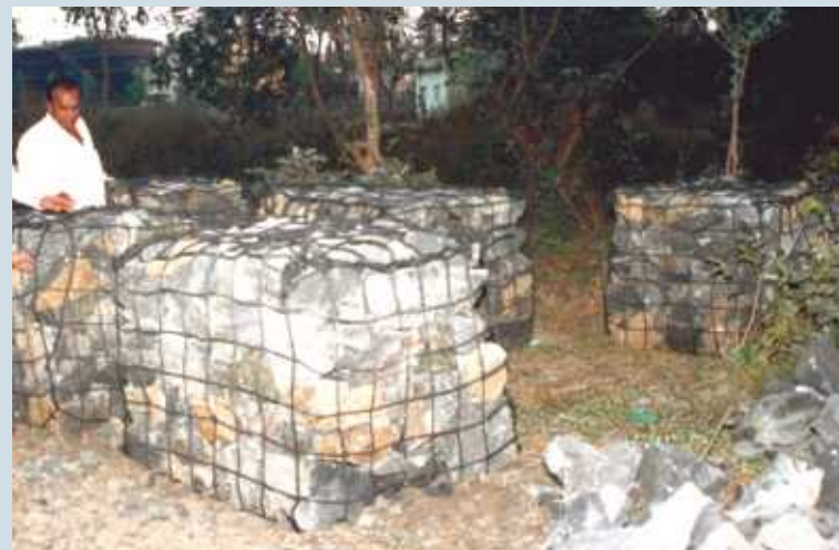
Filled Gabions ready for installation
