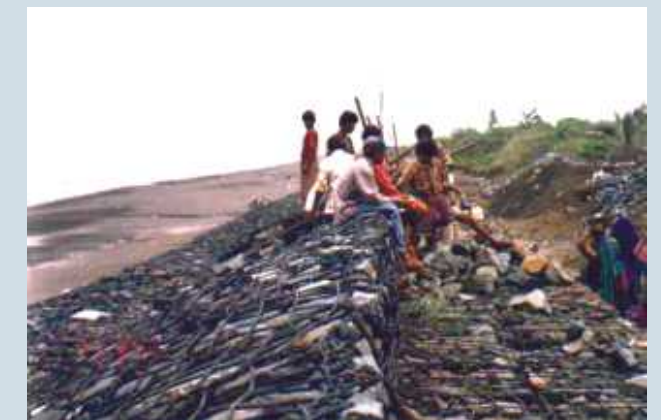
Top view of Gabion wall at Swaminarayan temple, Tithal
