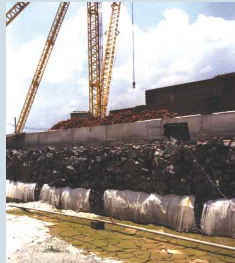
Gabion wall at Swaminarayan temple, Delhi
