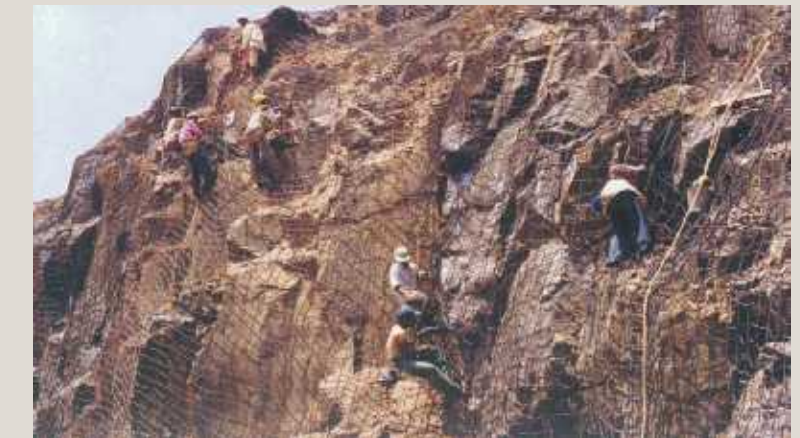
Polymer ropenet at Vilvade Cutting, KRCL
