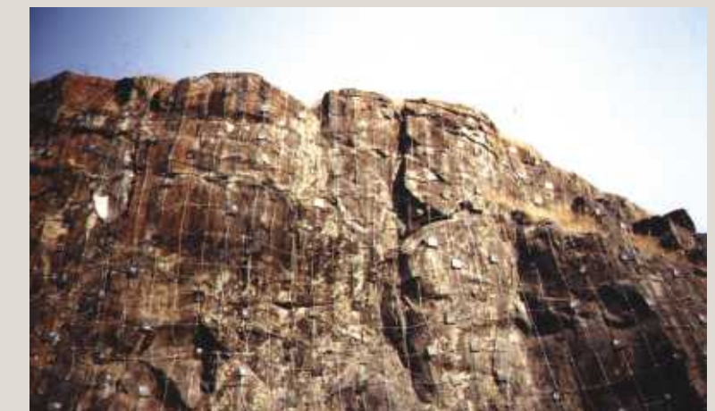
Steel wire ropenet at Ashti Cutting, KRCL
