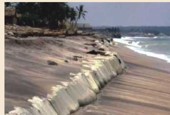
Geotextile filter wrapping erosion control wall at PWD, Tamilnadu site
