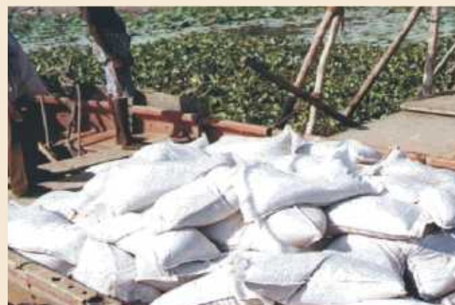
Geobags ready for installation at SMC, Surat
