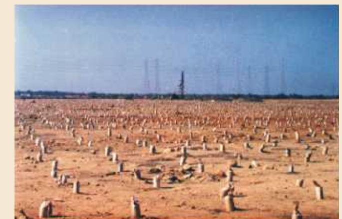
Encapsulated sand drains at MIDC, Thane
